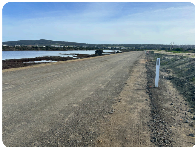
Reinstated Greyhound Road looking towards North Side Hill.
