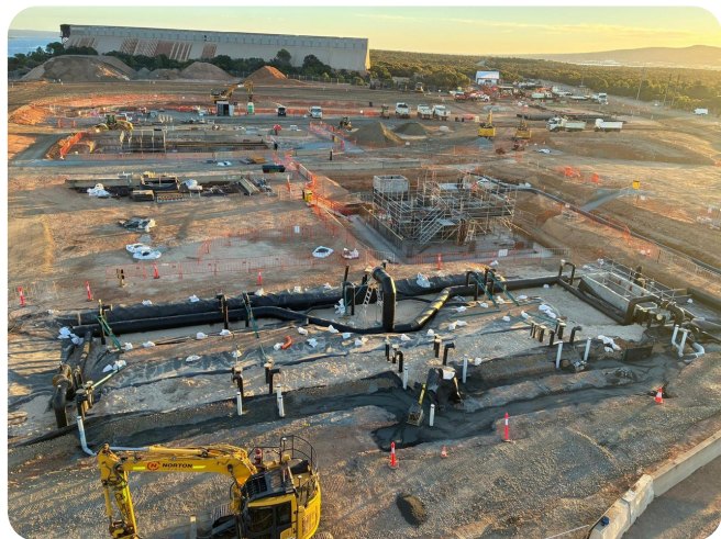
An aerial view of construction works on the desalination plant site.
