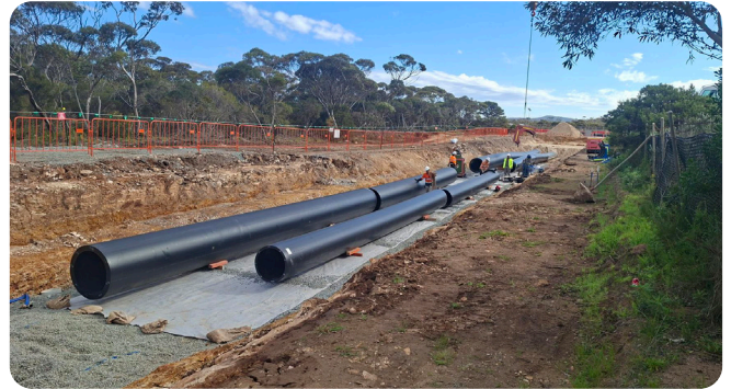
Terrestrial pipeline construction.
