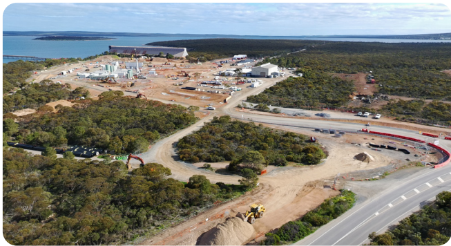
Aerial view of the desalination plant site.
