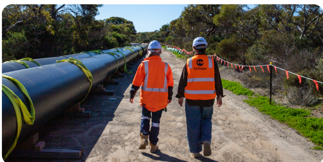
Pipes are ready for welding on land.
