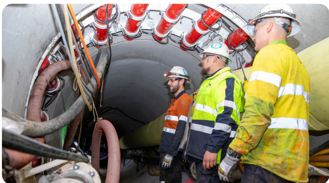
Work continues inside the tunnel under the seabed.
