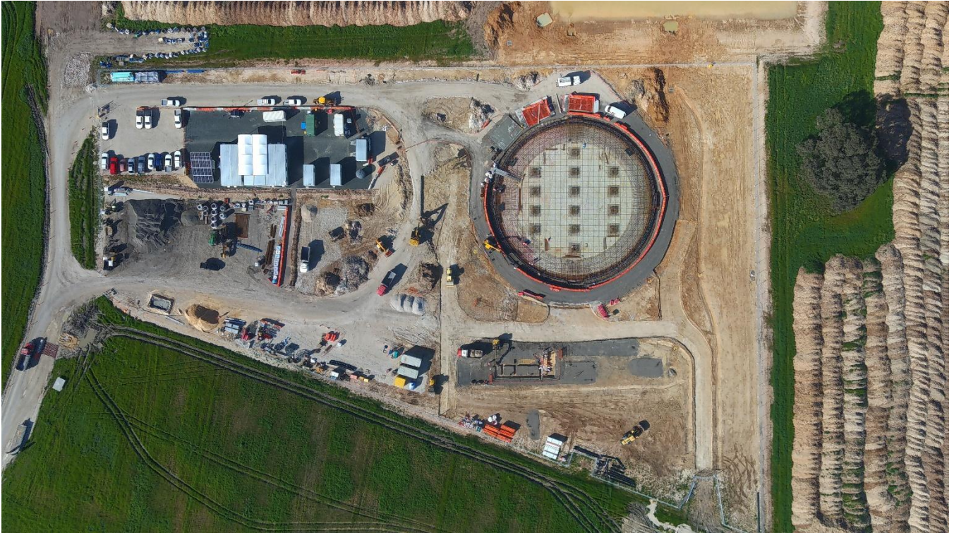
Site compound and construction area for the new 9- megalitre water storage tank
