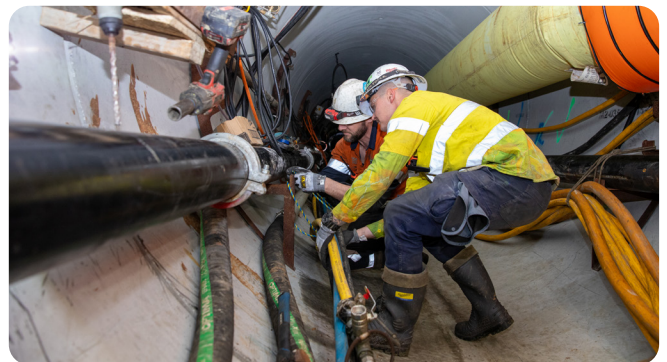
Work continues on the marine infrastructure.
