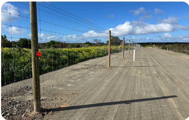
New fencing along Greyhound Road
