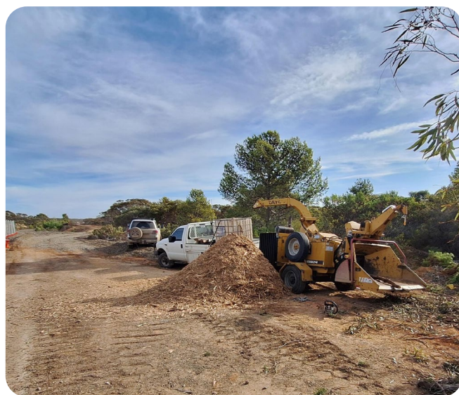
Vegetation clearing along transfer pipeline alignment
