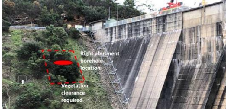
Drilling on right abutment
