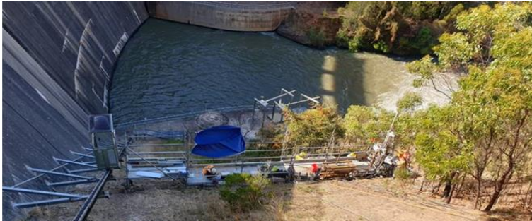
Drilling platform anchored in the right abutment
