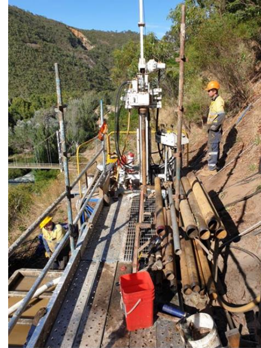
Drill rig in place on right abutment
