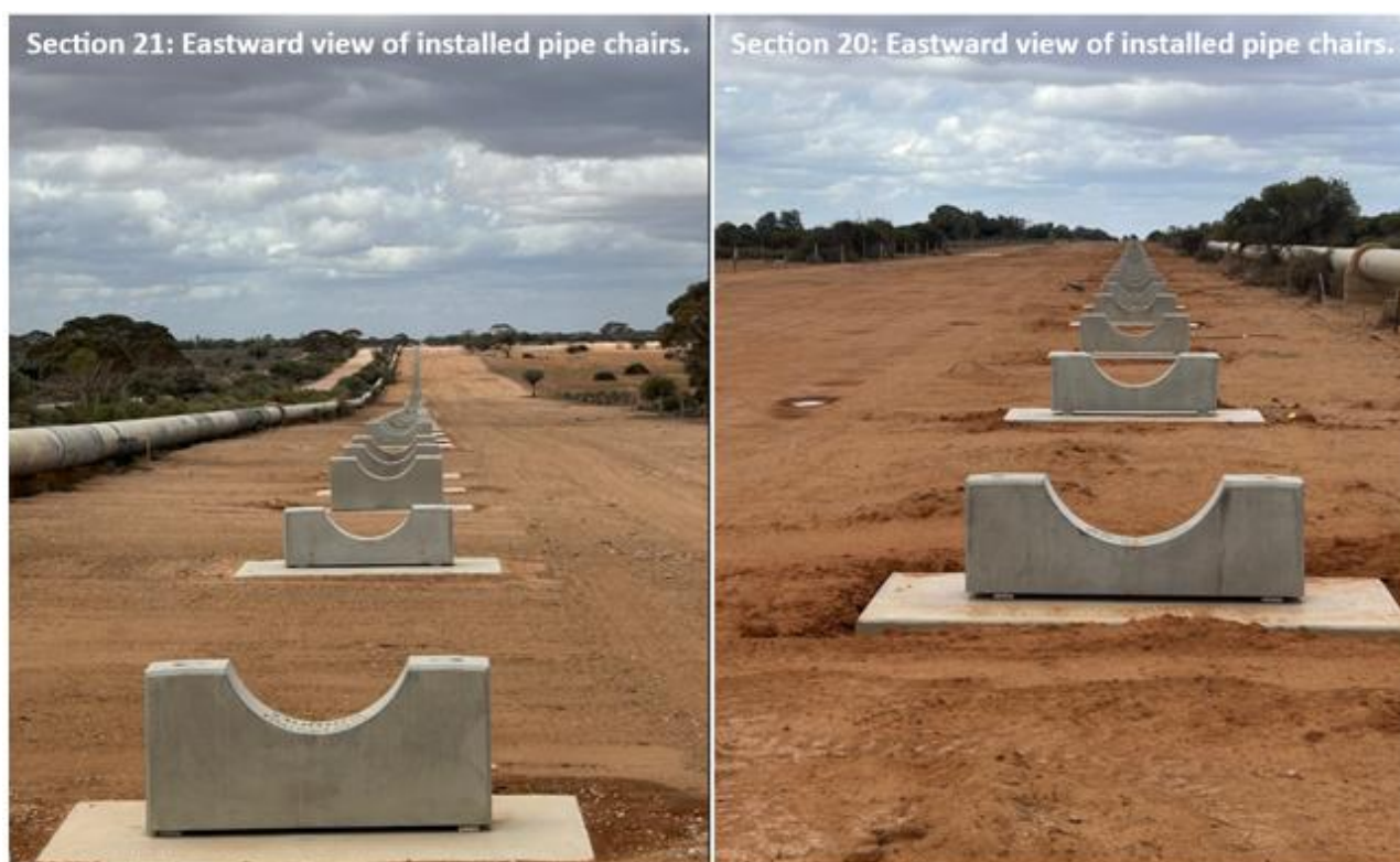
Figure 2 placement of pipeline support chairs, section 20 &amp; 21
