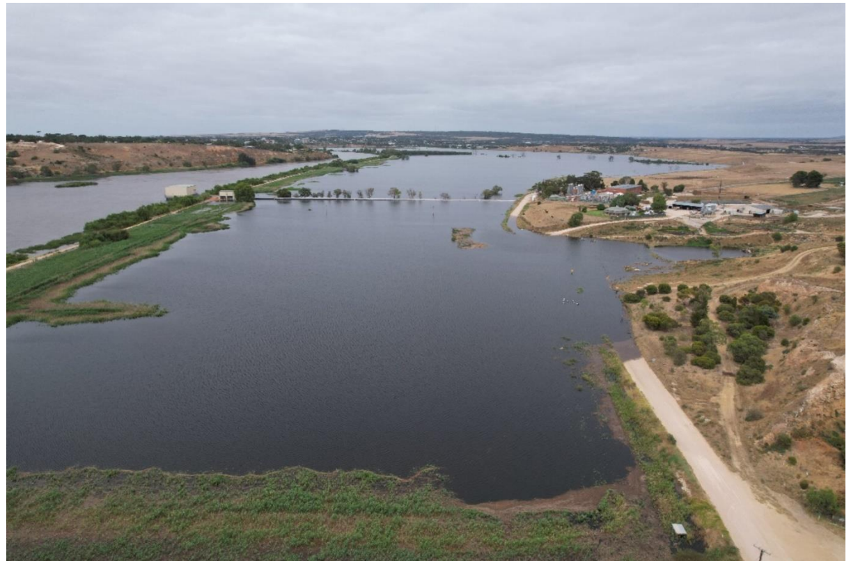
Southern end of Toora Irrigation Area looking towards Mobilong during flood. The SA Water drinking water supply offtake is shown on the left of the picture with the road to this infrastructure inundated along with the public road in the foreground
